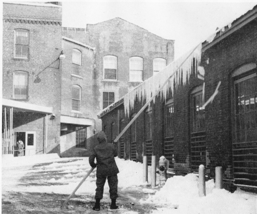
Here we have Patsy Pruscino, well-known yard maintenance man, performing an important safety work, following the recent snowfall and freeze. These icicles that formed on the edge of Wire Mill roof would be a grave danger to any person who ventured beneath them — say, a fireman at the fire plug.
